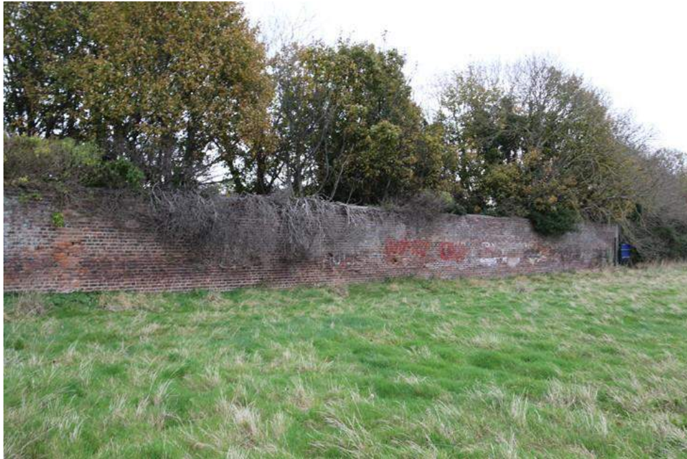
Figure 11-19 Brick-faced wall near the northern boundary
