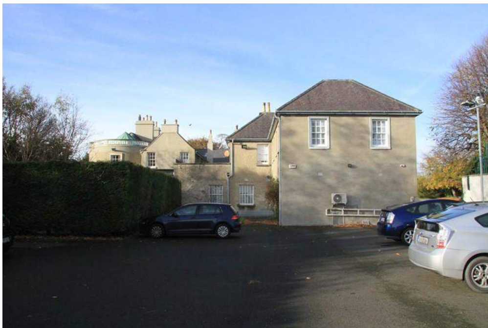
Figure 11-16 Eastern elevation of Sybil Hill House
