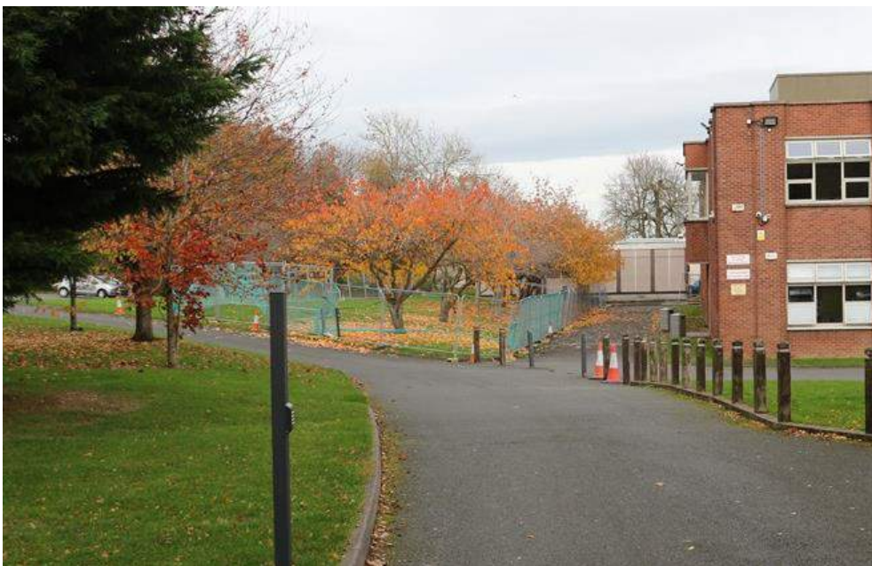
Figure 11-11 Site for proposed access, with St Paul's School to right and Sybil Hill House to left
