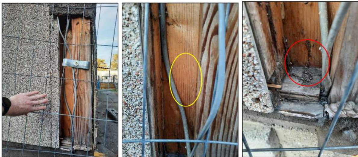
Figure 5-12 Images of the damage to pre-fab structure's south-western corner. Left-right: The damage, potential claw marks (Yellow) & insect remains at the base of the hole (Red).
