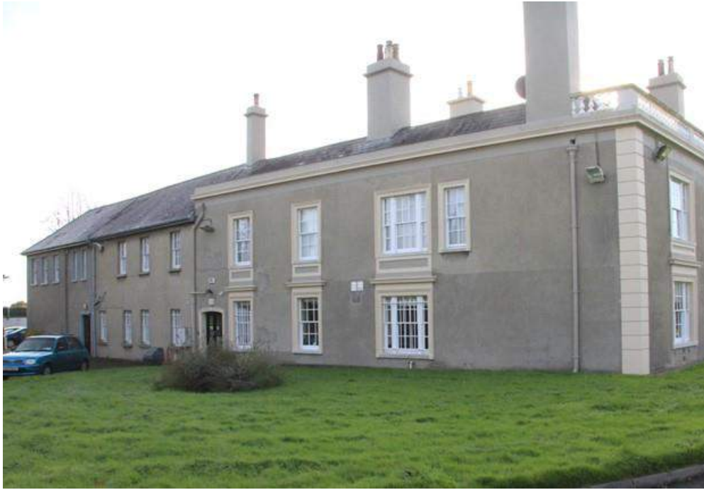
Figure 11-15 Northern elevation of Sybil Hill House
