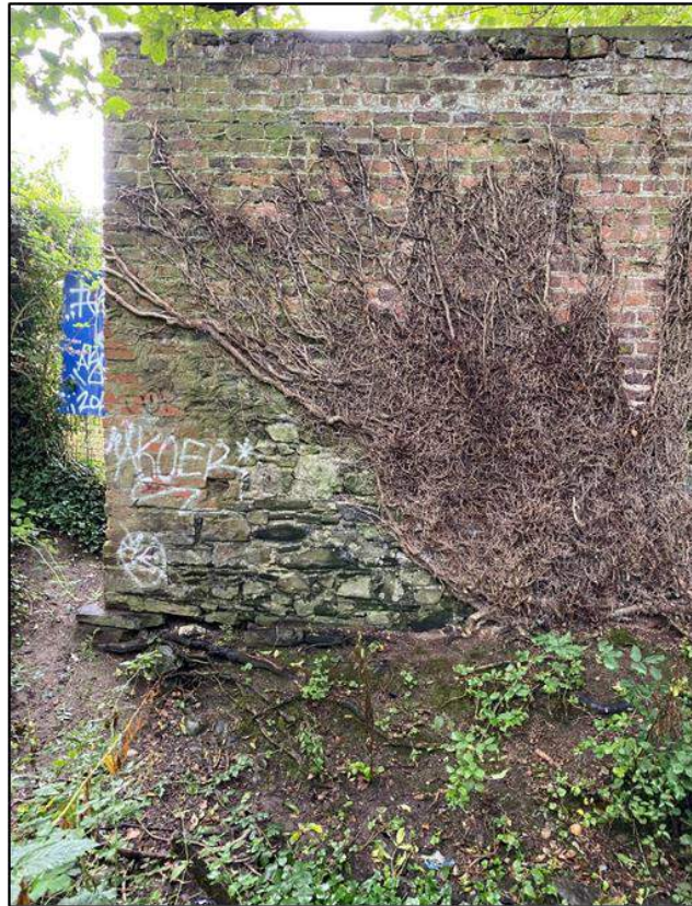
Figure 11-25 North facing elevation of Walled Garden wall, showing limestone foundation
